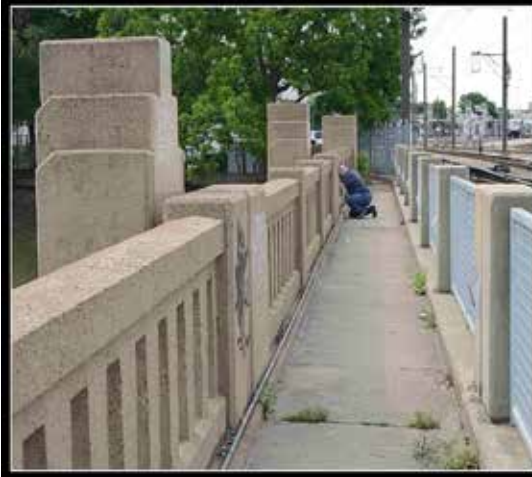
View looks west from atop the triple underpass
